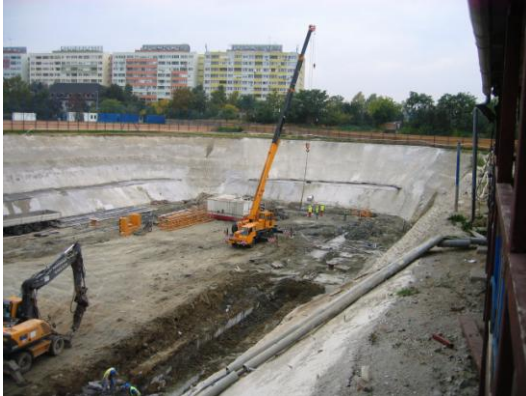
Open Cut Excavation Kelenfeld Station
