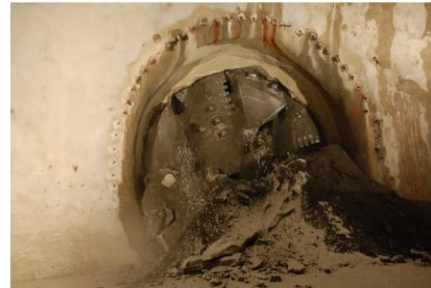
TBM Breakthrough
