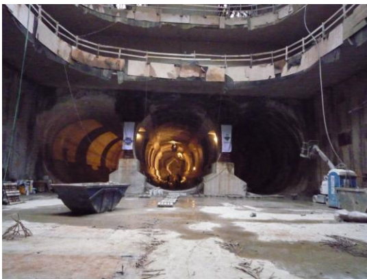
Staged SCL Construction at Rakozci Station
