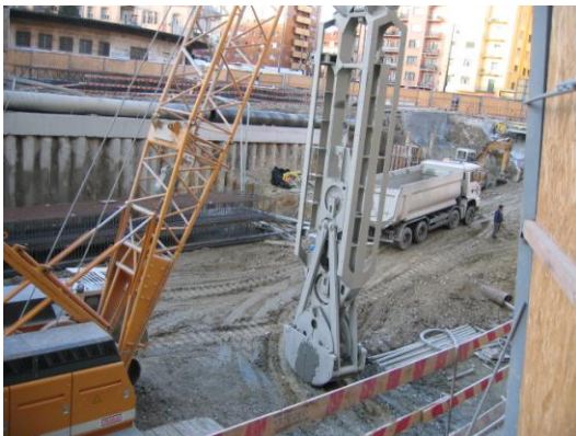
Piling and Diaphragm Wall Construction at Moricz Station
