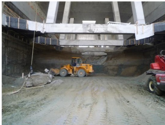
Framework Construction at Keleti Station
