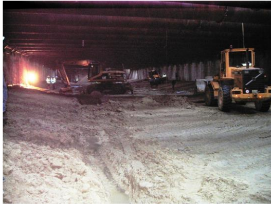
Open Cut Excavation Nepshinhaz Station
