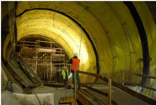
Platform Caverns SCL Construction at Gellert Station
