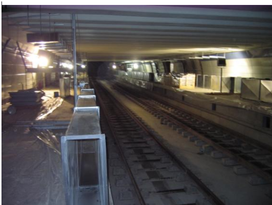
Fit Out of Station and Track Laying
