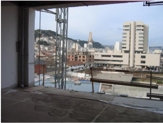
Central Control Facility under Construction
